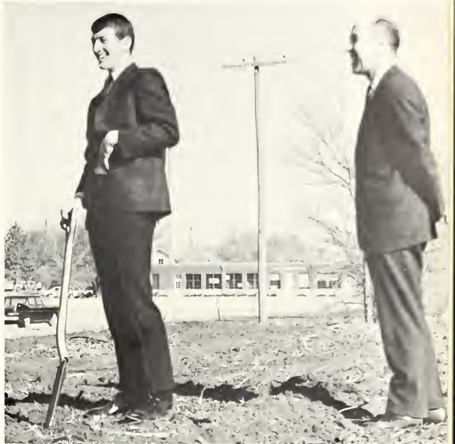
Jerry Hershberger, student representative, breaks ground for the new dorm while Merle Bender, director of development, looks on.
